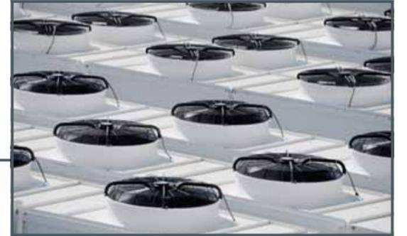
In the **condenser**, the heat is released from the refrigerant and transferred to the environment. The refrigerant vapour condenses due to heat dissipation. The refrigerant vapour must have a higher temperature than the environment. This required condensing temperature is directly proportional to the pressure generated by the compressor. Condensation takes place at constant high pressure.
