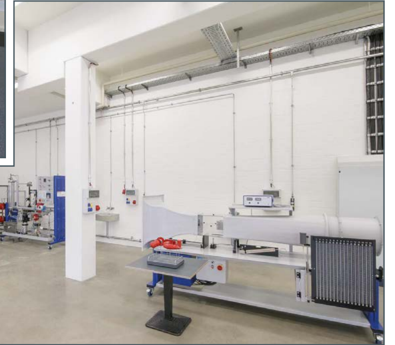
Exhibition of large training systems, ready for demonstration on the ground floor
